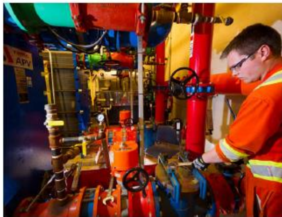
Cleaning the District Energy System heat exchanger strainers. Photo: Mike Crane
