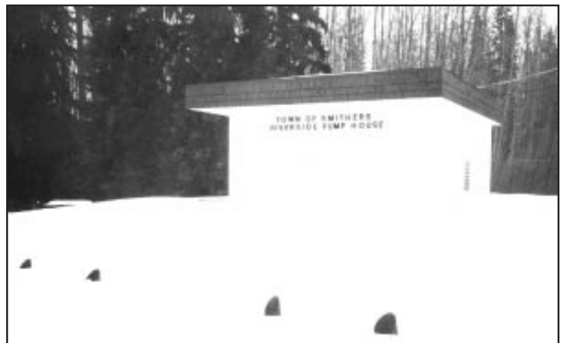
Winter view of Smithers' Water Pumphouse - Plant Profile continued on page 4.
