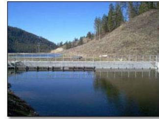
Pre-sedimentation Grit Pond
