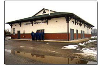
Enderby Water Treatment Plant
