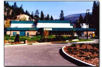
Penticton Water Treatment Plant
