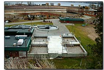
Summerland Wastewater Treatment Facility
