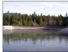
Backwash settling pond
