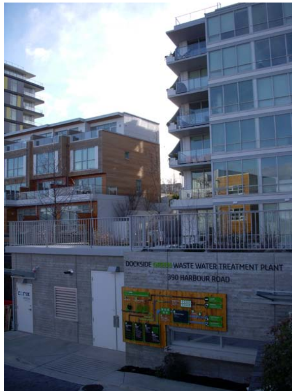
Figure - Dockside Green Wastewater Treatment Plant
