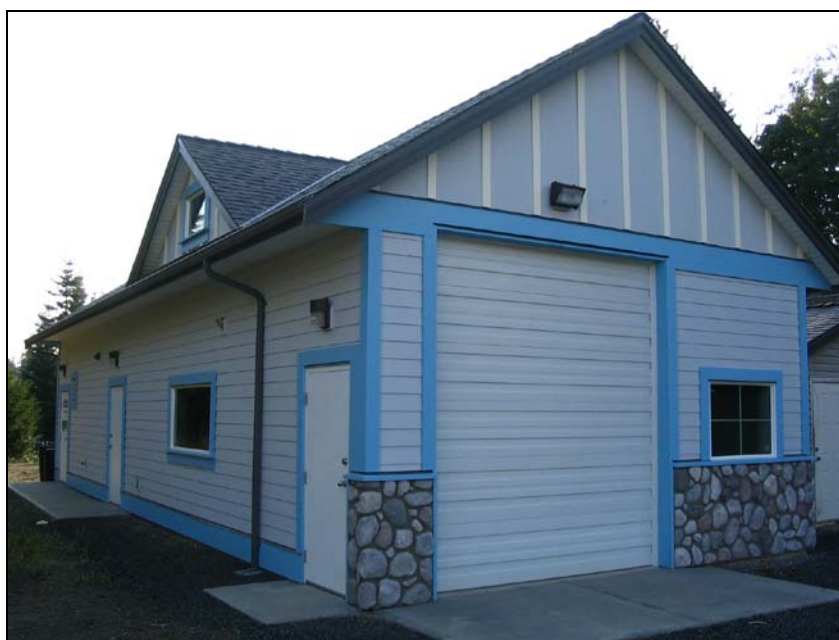
Drew Road Water Treatment Plant
