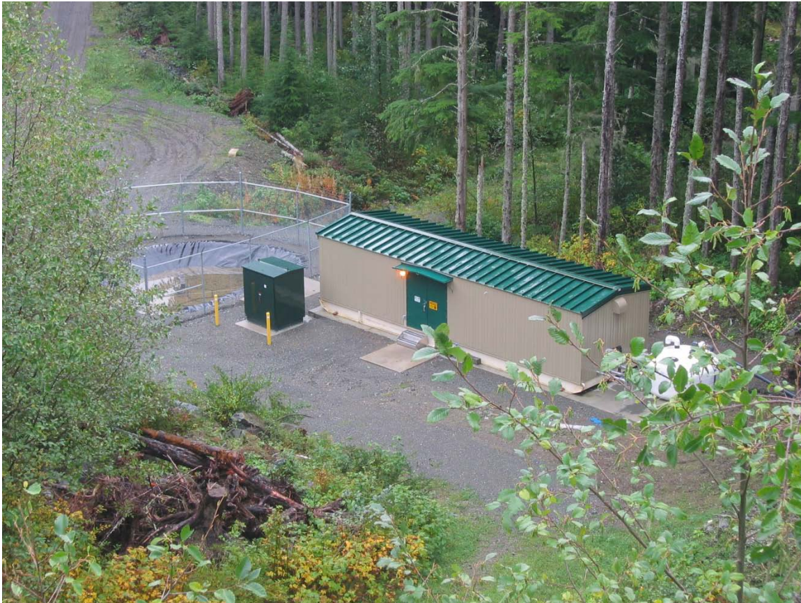
Water Treatment Facility
