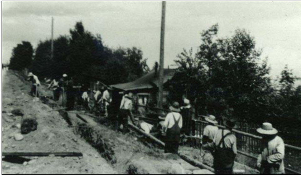
Chinese crew in 1947 laying pipe
