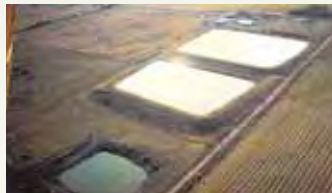
Trail Reservoir (80 Million US Gal.)
