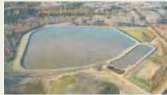
Hansen Reservoir (100 Million US Gal.)
