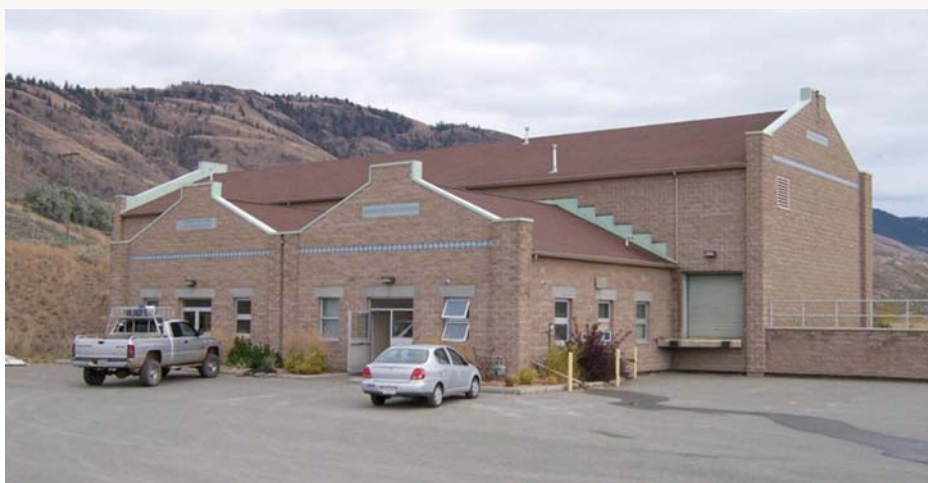
Tkemlups Indian Band Main Water Treatment Plant
