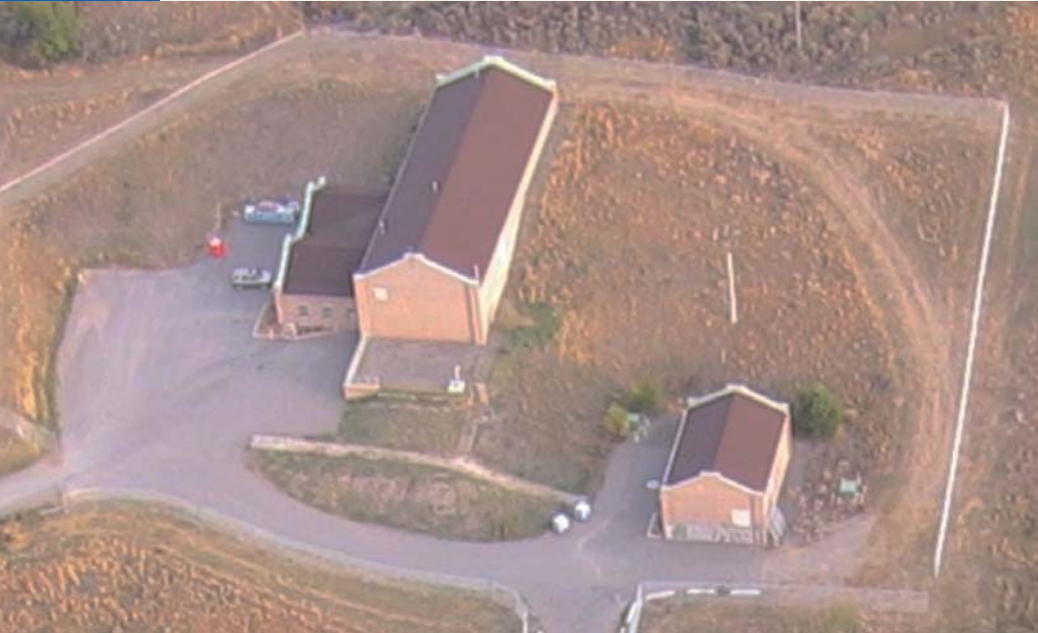
Aerial hot air balloon photo of Tkemplups Water Treatment Plant
