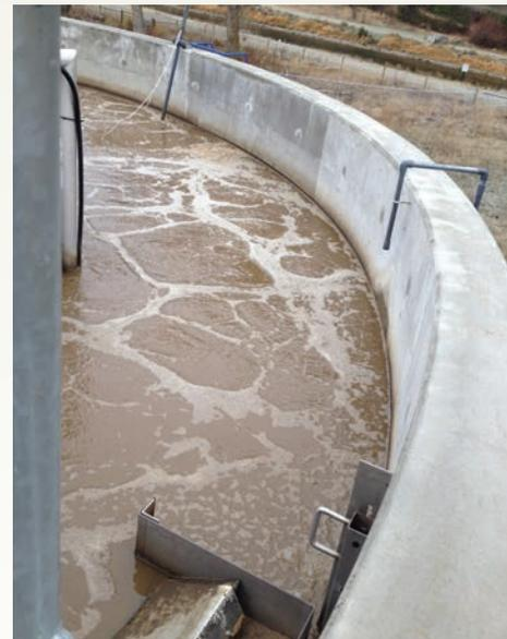
*Last Aerobic Zone with Alum Addition (Grey Drip Pipe) and Surface WAS (wasting) Box. Surface wasting has proven very helpful in resolving foaming and removing floating solids, leaves, etc. that find their way into the Bioreactor.*
